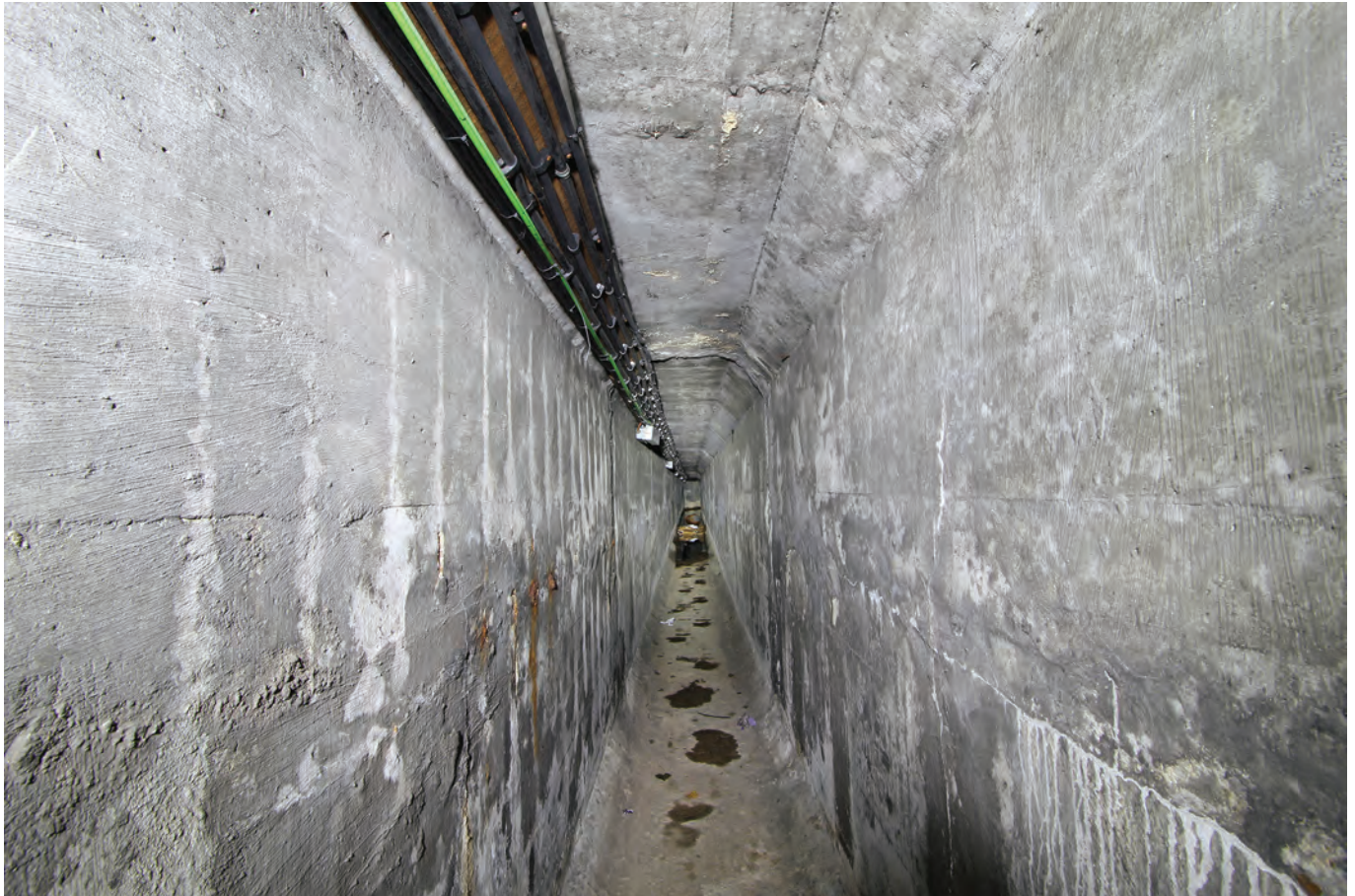
The emergency exit tunnel from the basement of Brent town hall
